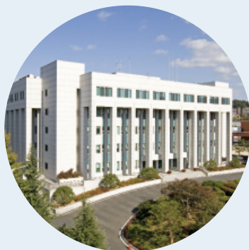
Woosong University's Administration Building
